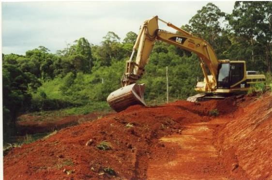
Operator cleaning bund batter for even soil profile. Makes for easier follow up management of site and good seed strike for cover crop to establish as soon as possible.
