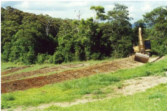
This photo shows a site being developed specifically for an orchard. The swales have been constructed in a way that the top swale, when full of water, drops excess to the left, into the swale below it. The second swale spills to the right into the third and so on. The water finally leaves this situation into a dam at the bottom of the site.
