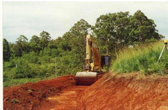
Note laser level on the right. Machine has laser pickup on boom for precise work. It is fundamentally important that the swale is constructed precisely level.
