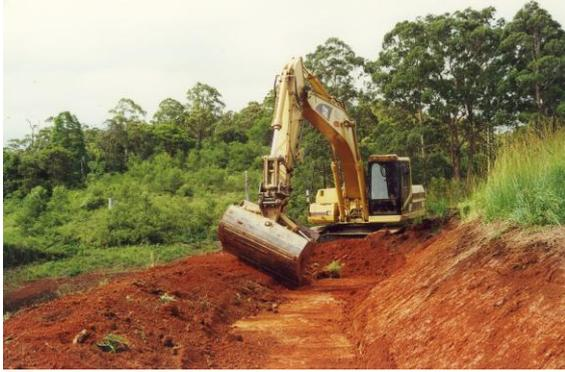
The operator here, is cleaning up the inside bund batter. This is very important as there will be approx 400mm of free board on this batter when the swale is full of water.
