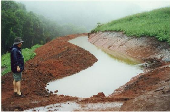
Approx 5 days after construction. Note that just to the right of the person is where very specific height excavations have been made for the spill way. This swale has an average freeboard of approx 400mm then spills at that level into a spoon drain which is directed to the next swale down.
