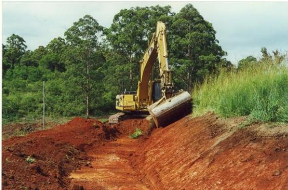
Swale being constructed on a steep slope in high rainfall area. Good batters allow for ease of access over site and better blend into natural landscape. You can comfortably use this swale for tractor access over site. Annual ripping is promoted for vehicle access situations.
