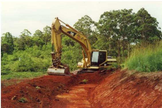
Operator is setting level for the top of the bund using laser pickup on his boom.
