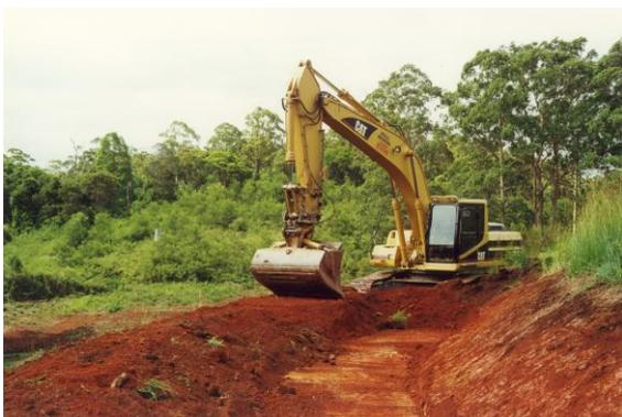
When level is set, operator then puts on the final finish, to the precise set level on the top of the bund.
